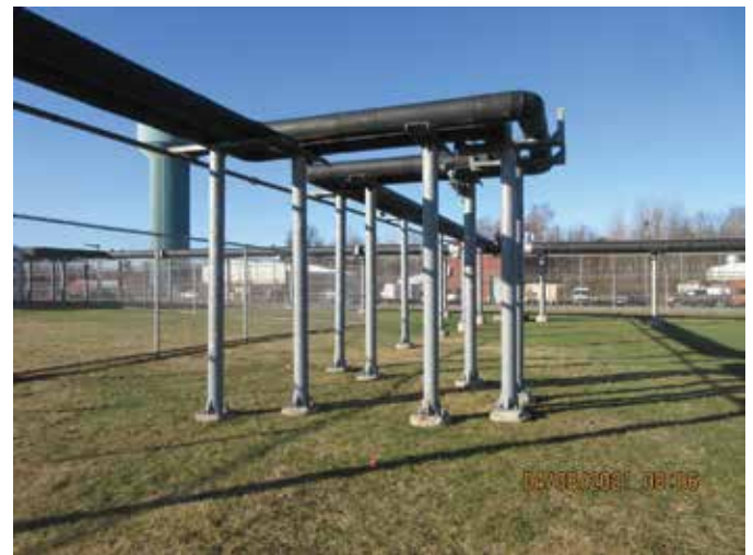
Rehabilitate Exterior Heating System Stanchion Supports, Gouverneur Correctional Facility
