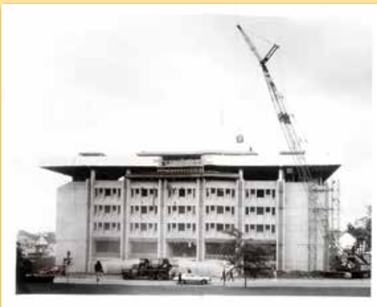
SU Bird Library. Under construction. Syracuse, NY 1971
