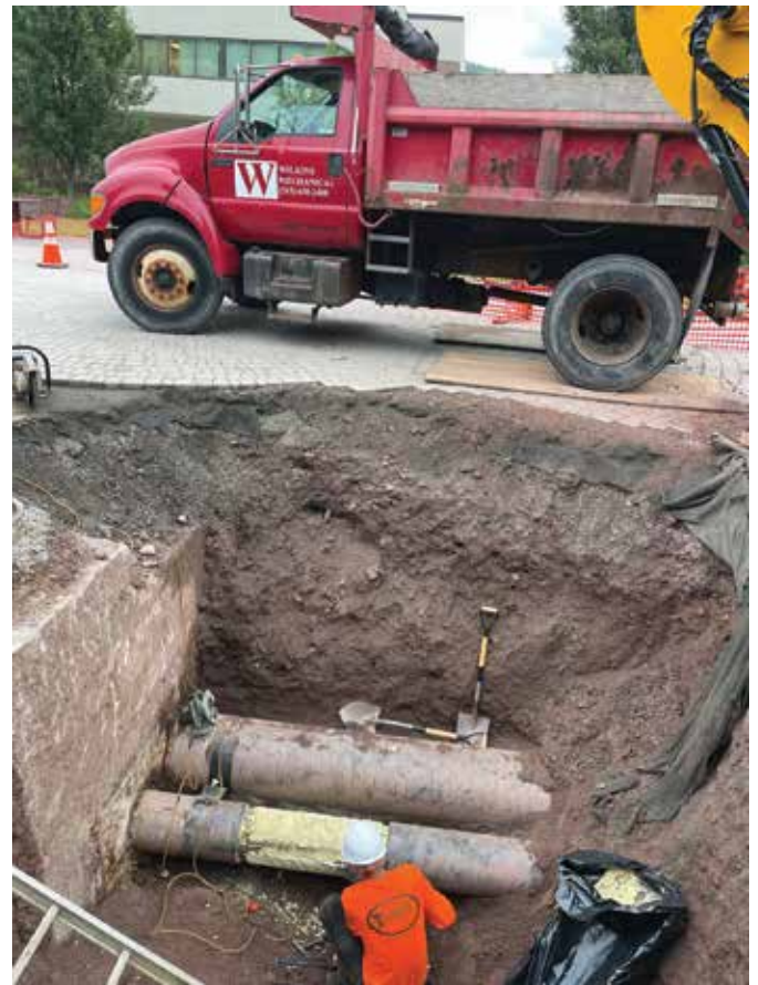
Condensate Repair Manhole #3, Farrell Hall SUNY Delhi
