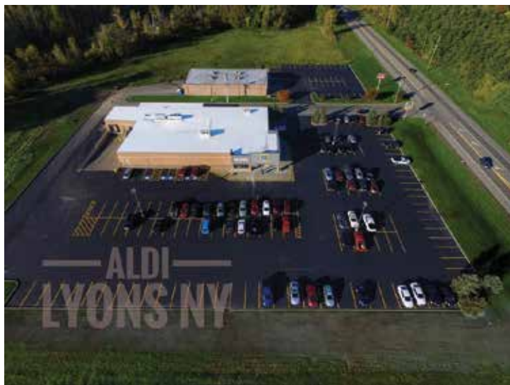
J&B project at Aldi in Lyons, NY
