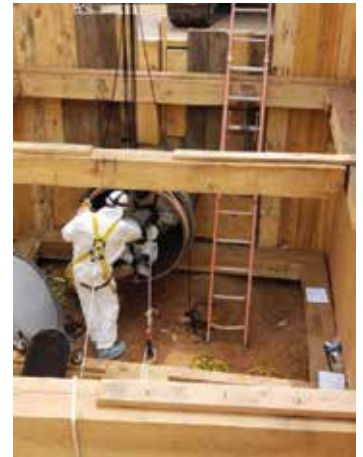
Camden Group works on piping for PSE&G
