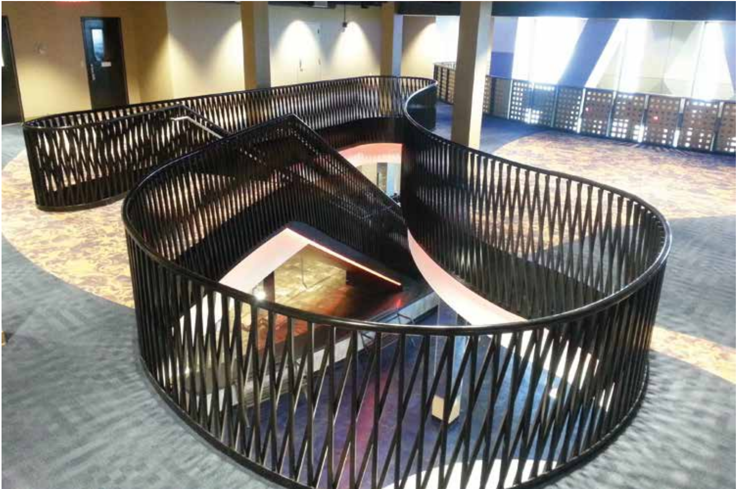
Curved stair, rails and structural opening at Batavia Downs Casino. This work was completely designed, detailed, fabricated and installed by staff members of Mattessich Ironworks.
