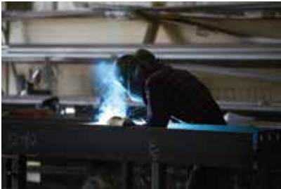
Welder/fabricator Gary Durant, a Navy veteran, details a beam bound for the East Lake Commons project in Oswego.
