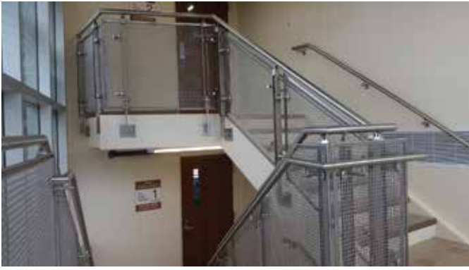
A four-level tube steel stair with stainless steel mesh rails designed in collaboration with the architect at SUNY Brockport's Lathrop Neff hall addition.
