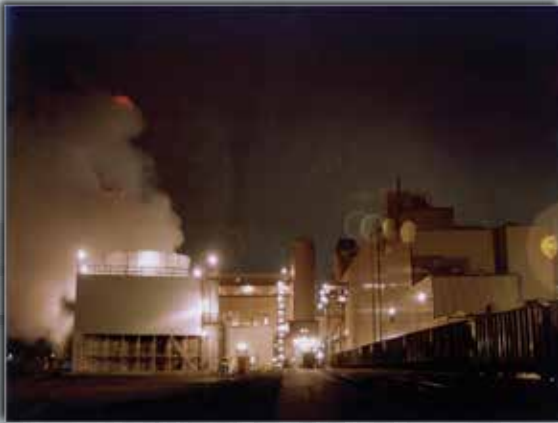
Hydroco CoGen Plant, Solvay NY. c1990 - GM Crisalli & Associates was the General Contractor for the Administration Building and Construction Manager for numerous other projects at the job site.
