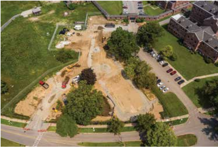
VA Medical Center, Parking Lot Expansion. Montrose, NY.
