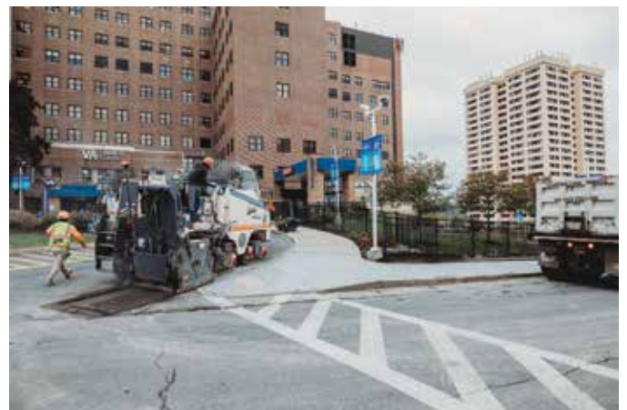
VA Medical Center, Sidewalks and Accessway Renovation. Syracuse, NY.
