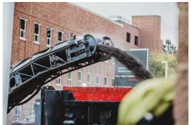
Construction Working Photos
